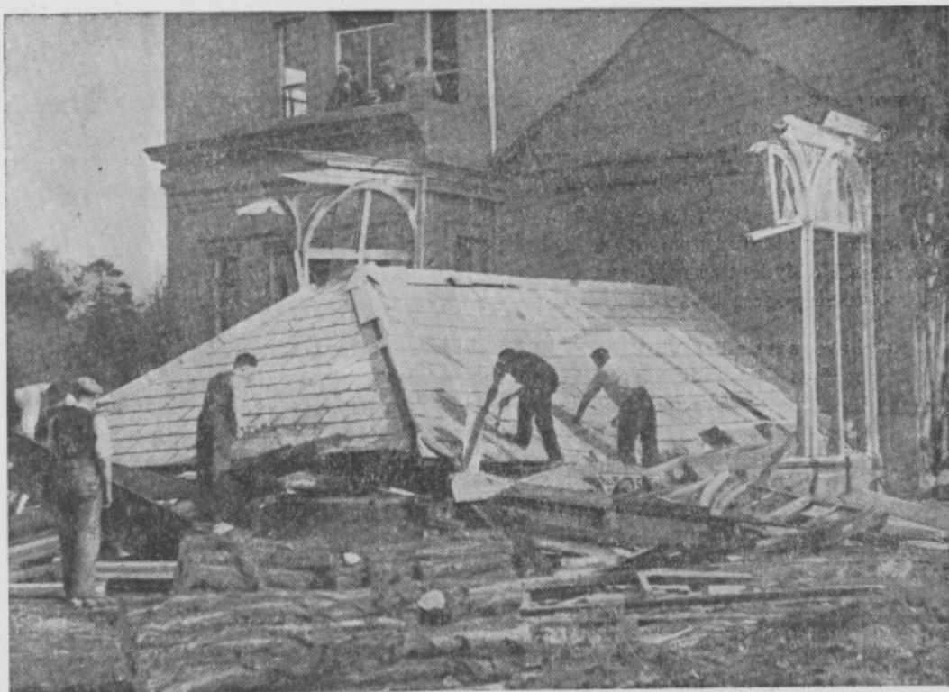
The Demolition of the Old Conservatory
